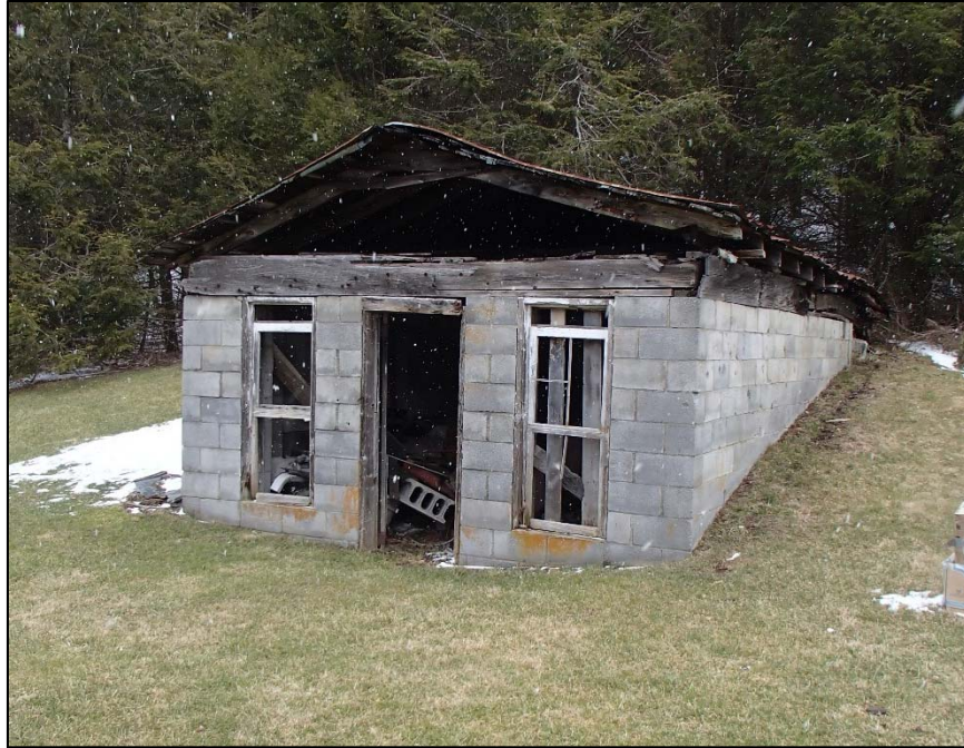
Figure 34: concrete block outbuilding, southwest corner
