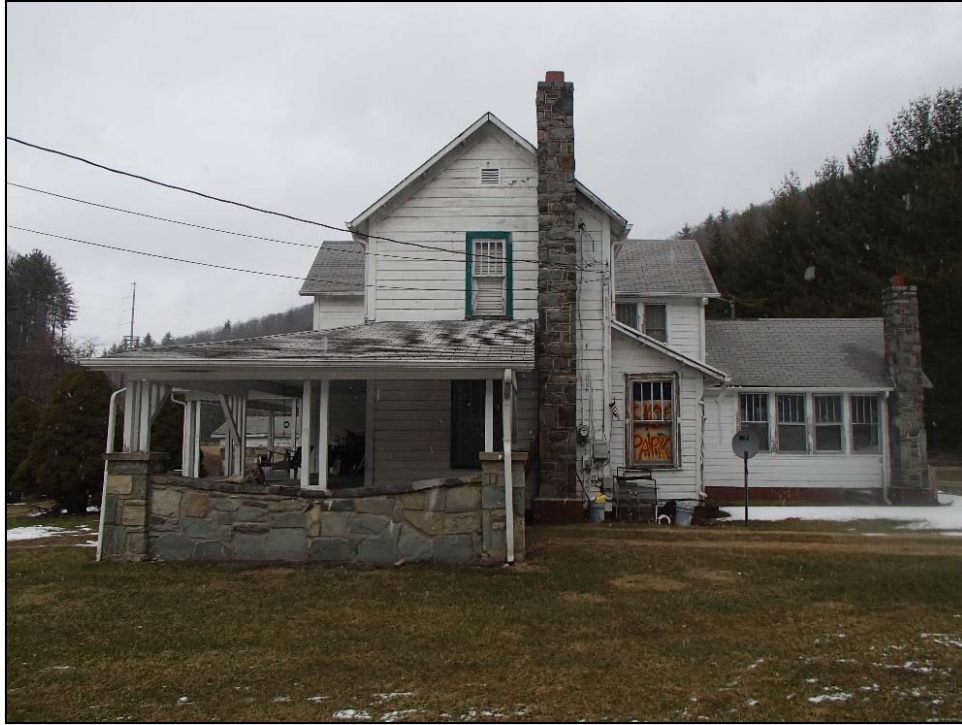
Figure 28: Shull House, south elevation
