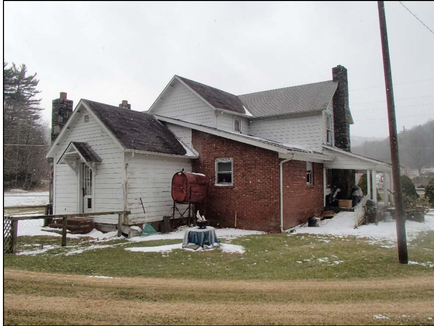
Figure 30: Shull House, northeast corner
