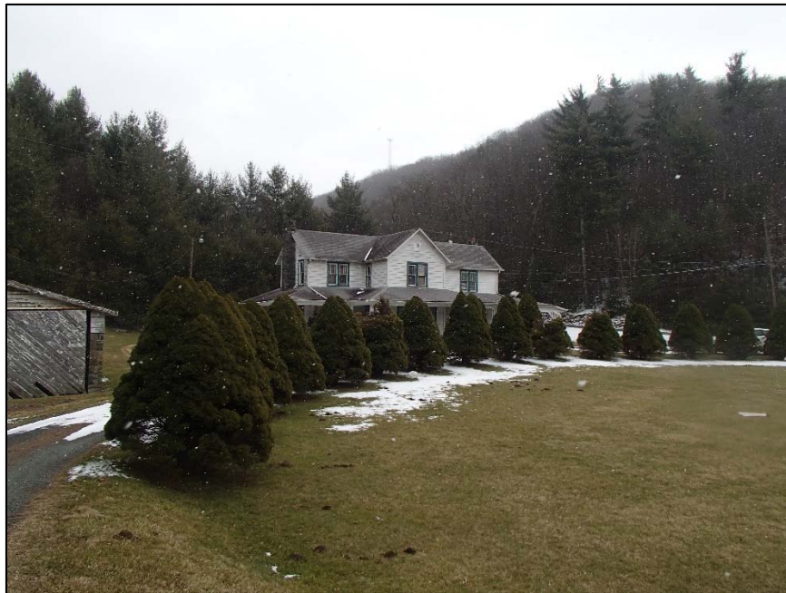
Figure 37: Shull House, west elevation from U. S. Highway 321
