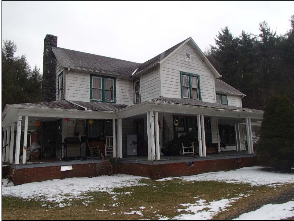
Figure 26: Shull House, west elevation
