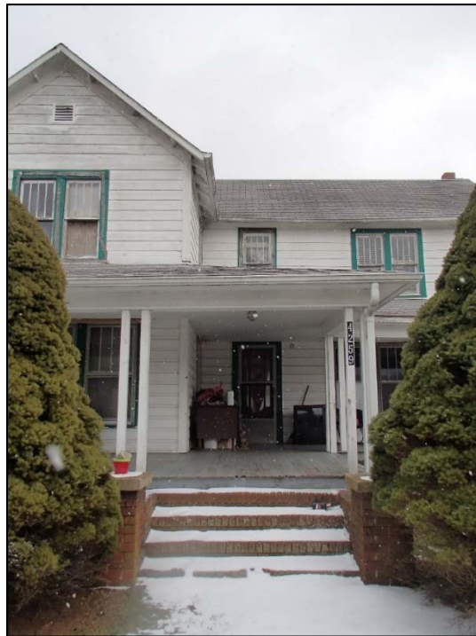
Figure 27: Shull House, west elevation, front door
