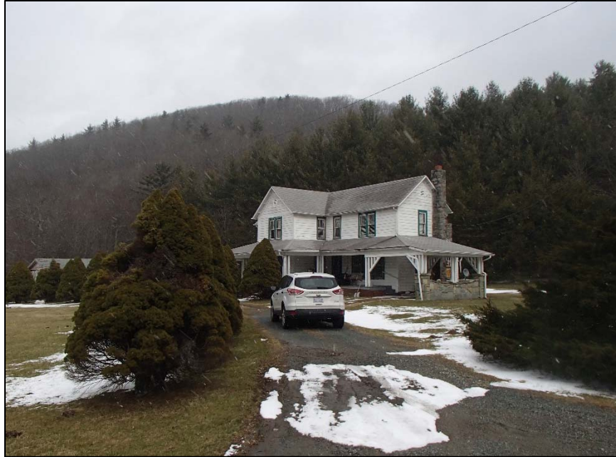
Figure 36: Shull House, southwest corner
