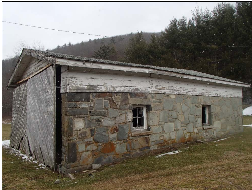
Figure 33: stone outbuilding, southwest corner
