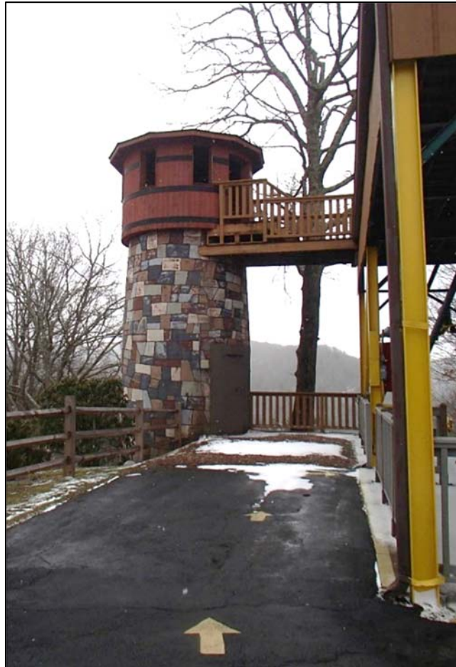
Figure 14: Miner's Mountain Chairlift, upper level with a castle turret converted to a water tower
