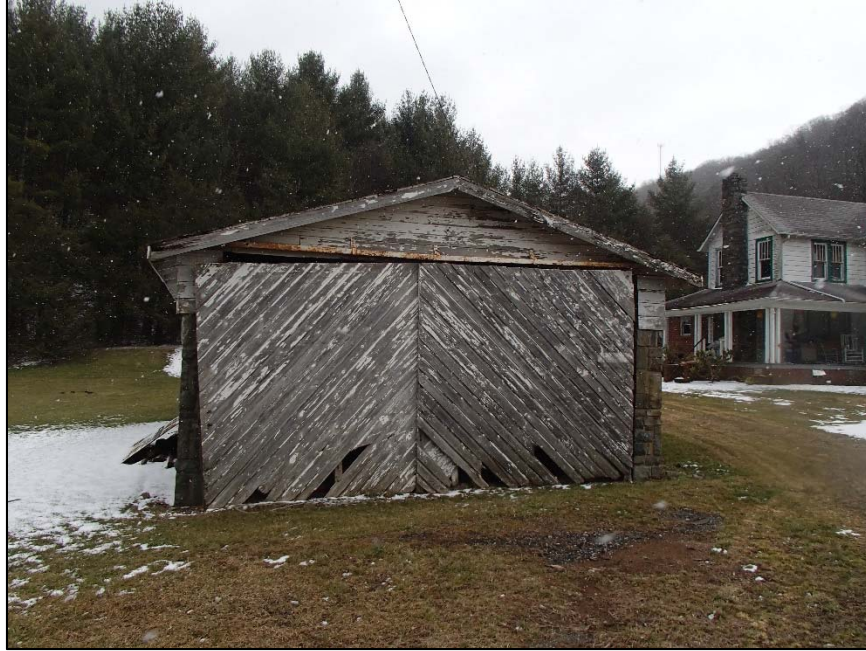
Figure 32: stone outbuilding, west elevation
